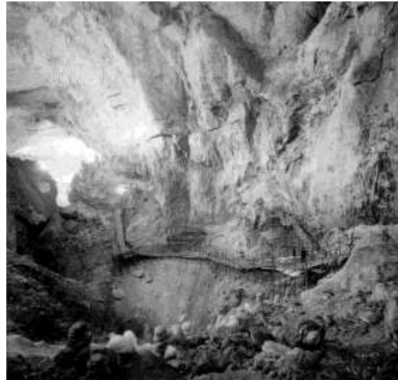
Figure 8: During the works in the Upper Galleries in 1967.
